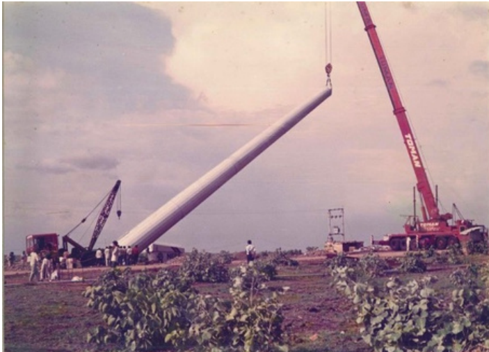
Jamgodrani Hills, Madhya Pradesh, 13MW
